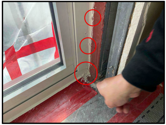
FIGURE 8 - Unit 1000 - View of sealant joints to be removed and replaced at not cleanly tooled locations.
