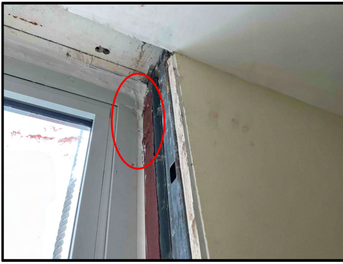
FIGURE 7 - Unit 1000 - View of sealant joints to be removed and replaced at not cleanly tooled locations.
