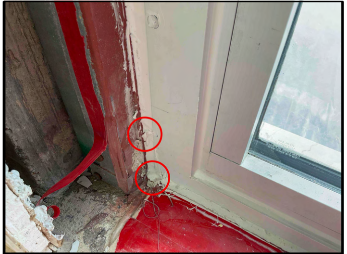
FIGURE 10 - Unit 1100 - View of sealant joints to be removed and replaced at not cleanly tooled locations.
