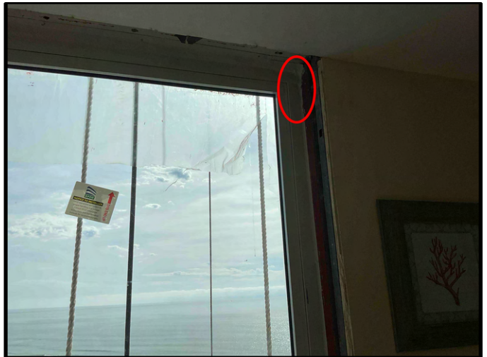
FIGURE 6 - Unit 1000 - View of sealant joints to be removed and replaced at not cleanly tooled locations.
