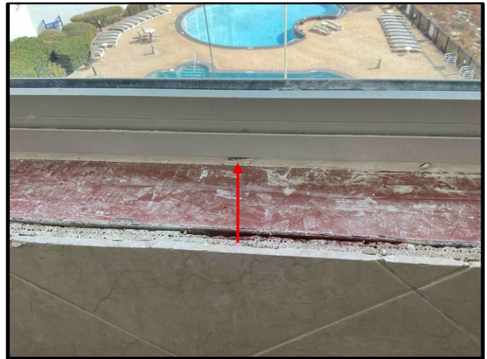
FIGURE 13 - Unit 500 - Northmost Bathroom - View of sealant joints to be touched up where void exists.
