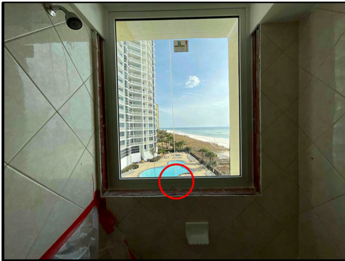
FIGURE 12 - Unit 500 - Northmost Bathroom - View of sealant joints to be touched up where void exists.
