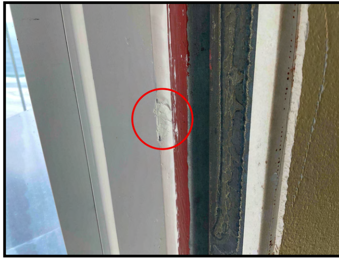
FIGURE 11 - Unit 1100 - View of sealant joints to be removed and replaced at not cleanly tooled locations.
