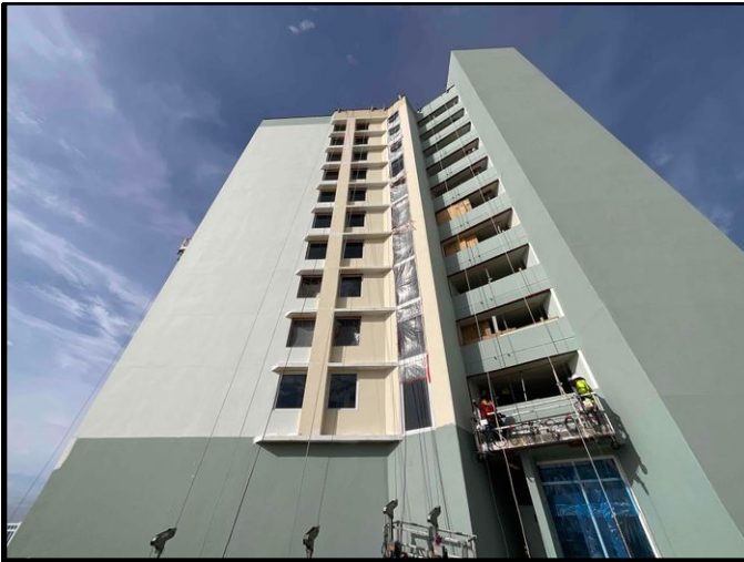
FIGURE 1 - East Elevation - Overall view of window replacement - Work in Progress.
