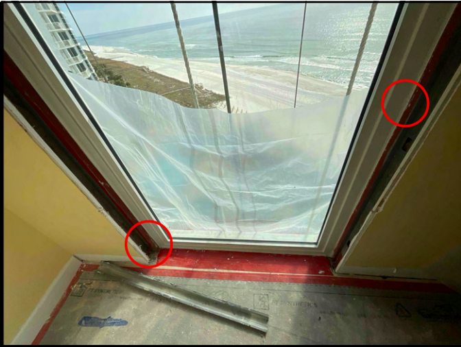
FIGURE 9 - Unit 1100 - View of sealant joints to be removed and replaced at not cleanly tooled locations.
