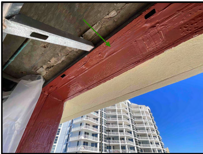
FIGURE 7 - Unit No. 1100 - Bathroom - View of new FastFlash waterproofing installed at rough opening.
