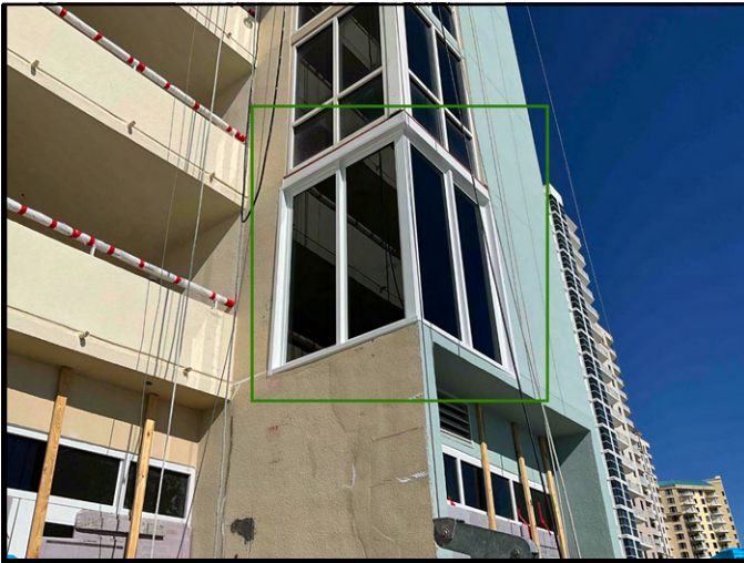
FIGURE 1 - Unit No. 200 - South Bedroom - Overall view of mock-up EFCO Series 2701 Fixed Window at corner condition.
