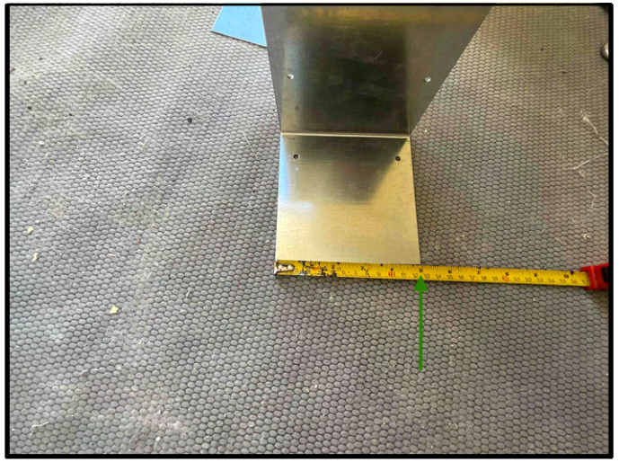
FIGURE 6 - Unit No. 1100 - North Bedroom - View of EFCO window clip measured at the required 5".
