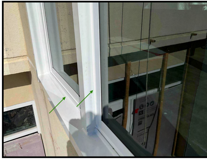
FIGURE 3 - Unit No. 200 - South Bedroom - View of sealant in good condition.
