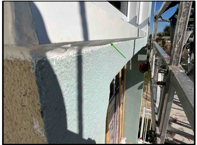
FIGURE 2 - Unit No. 200 - South Bedroom - View of sealant in good condition.
