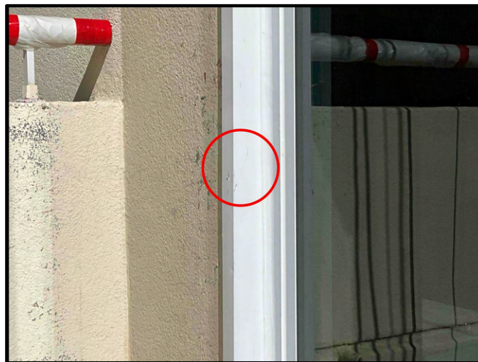
FIGURE 4 - Unit No. 200 - South Bedroom - View of isolated damage to window frame. This was discussed with the contractor on site and is to be touched up with additional paint.
