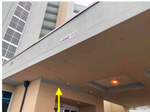
Photo 10 North Elevation - View of finish repairs at stucco - Work in progress.
