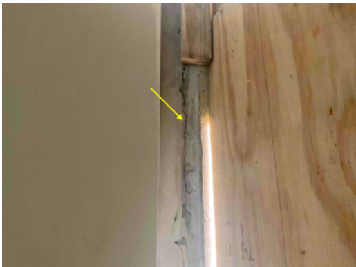
Photo 6 East Elevation - Lobby Storefront Window - View of hollow concrete at jambs of window rough opening - Work in Progress.
