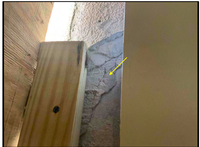
FIGURE 2 - Lobby East Elevation Storefront Window - View of hollow concrete at jambs of window rough opening - Work in Progress.
