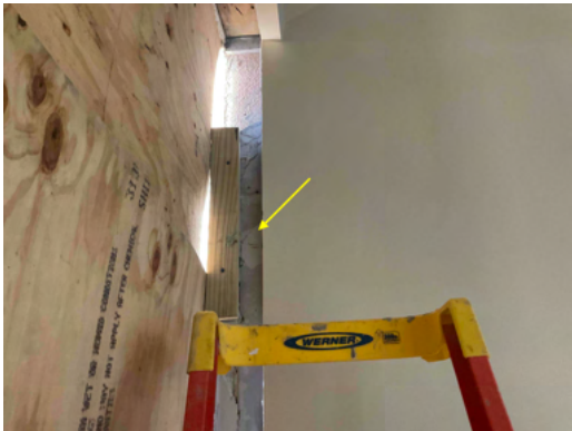
Photo 5 East Elevation - Lobby Storefront Window - View of hollow concrete at jambs of window rough opening - Work in Progress.
