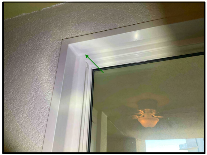
FIGURE 6 - Unit No. 802 - View of new PGT SH5500 Window in overall good condition.
