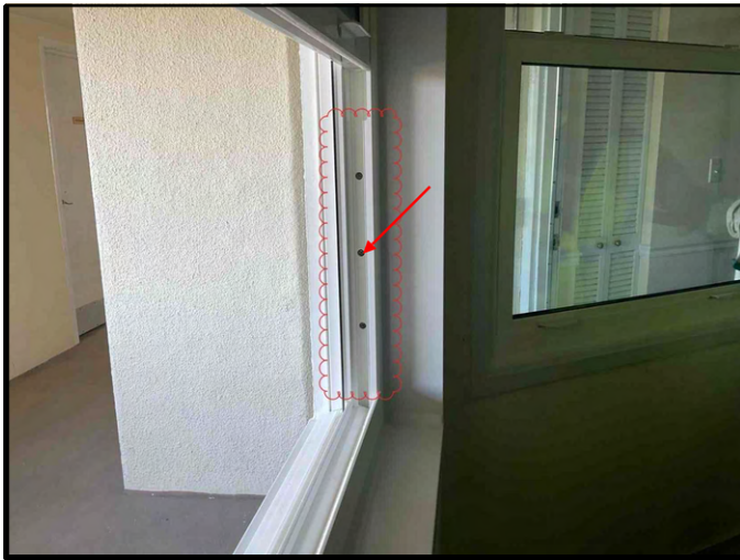
FIGURE 9 - Unit No. 204 - View of missing button caps - Punch Item.
