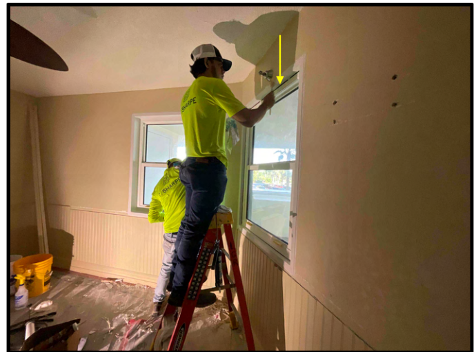
FIGURE 12 - Unit No. 112 - View of crew member installing sealant - Punch Item.
