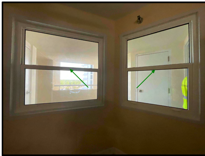
FIGURE 7 - Unit No. 702 - View of new PGT SH5500 Window in overall good condition.
