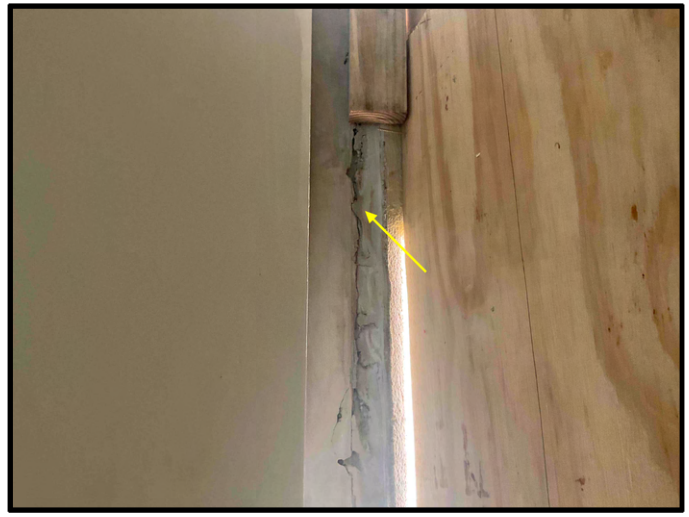
FIGURE 4 - Lobby East Elevation Storefront Window - View of hollow concrete at jambs of window rough opening - Work in Progress.
