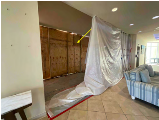
Photo 3 East Elevation - Lobby Storefront Window - View of plywood installed to protect opening during rough opening preparation - Work in Progress.
