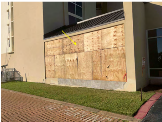
Photo 2 East Elevation - Lobby Storefront Window - View of plywood installed to protect opening during rough opening preparation - Work in Progress.
