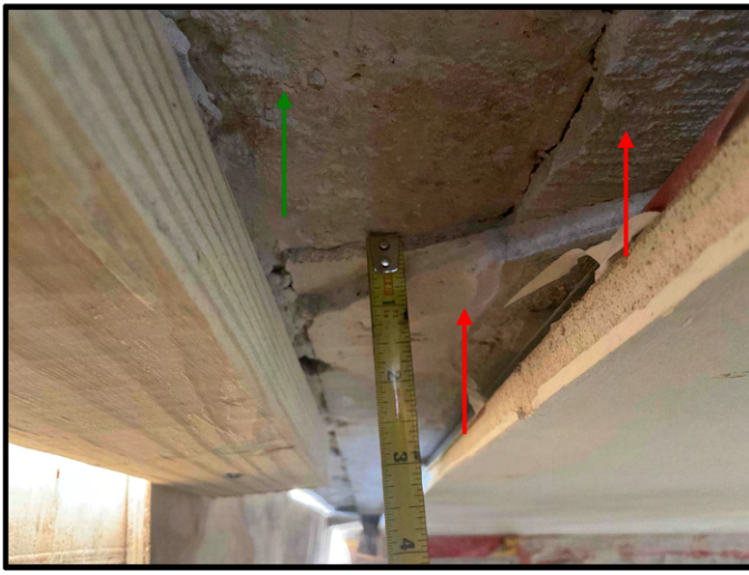
FIGURE 3 - Lobby East Elevation Storefront Window - View of hollow concrete at jambs of window rough opening - Work in Progress.
