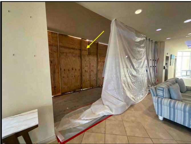
FIGURE 1 - Lobby East Elevation Storefront Window - View of plywood installed to protect opening during rough opening preparation - Work in Progress.
