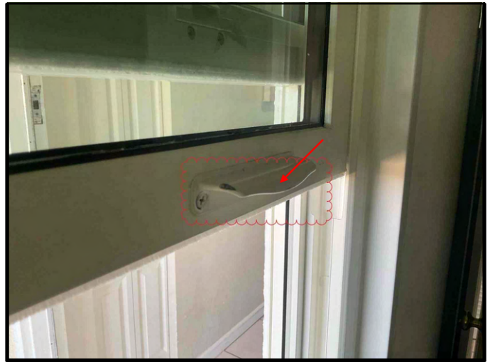
FIGURE 10 - Unit No. 304 - View of handle to be replaced - Punch Item.
