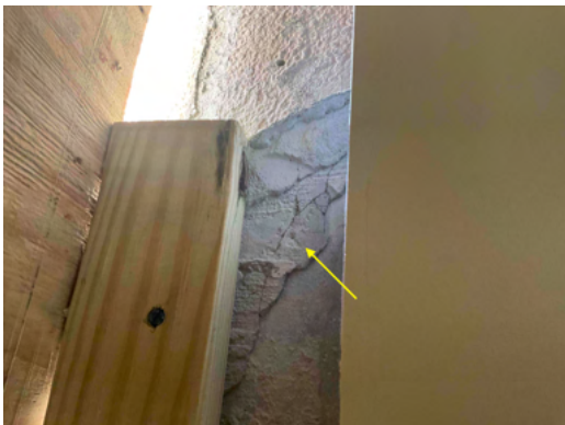
Photo 4 East Elevation - Lobby Storefront Window - View of hollow concrete at jambs of window rough opening - Work in Progress.
