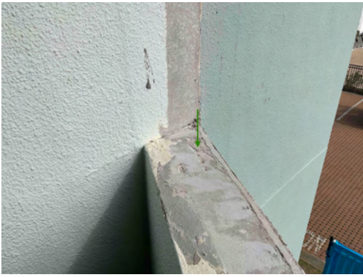
Photo 19 2nd Floor - View of concrete sill before waterproofing application.
