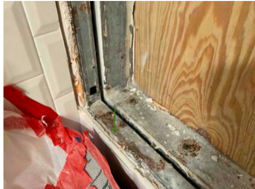
Photo 16 Unit No. 200 - View of existing tile removed from rough opening.
