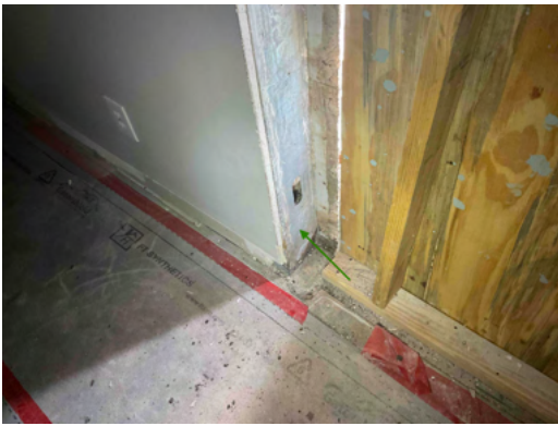
Photo 3 Unit No. 200 - View of metal framing moved inwards for window installation.
