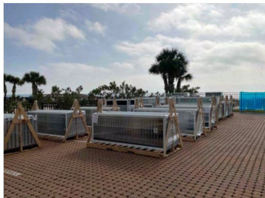
Photo 24 East Elevation - View of new EFCO windows stored on-site.
