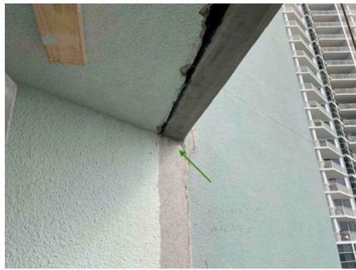
Photo 20 2nd Floor - View of stucco finish applied at new header framing.
