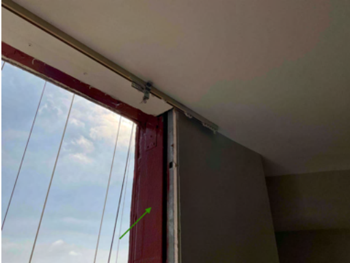
Photo 15 Unit No. 200 - View of new FastFlash waterproofing installed at rough opening.
