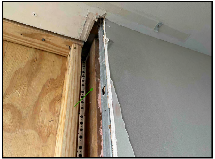
FIGURE 8 - Unit No. 200 - View of wood bucking at West Jamb.
