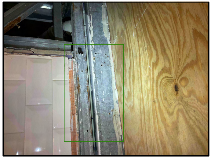
FIGURE 4 - Unit No. 200 - View of existing tile removed from rough opening.
