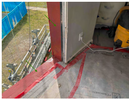
Photo 14 Unit No. 200 - View of new FastFlash waterproofing installed at rough opening.
