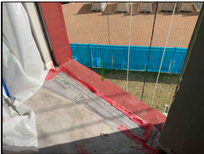
FIGURE 1 - Unit No. 200 - View of new FastFlash waterproofing installed at rough opening.
