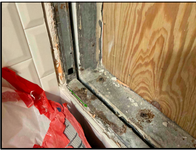
FIGURE 3 - Unit No. 200 - View of existing tile removed from rough opening.
