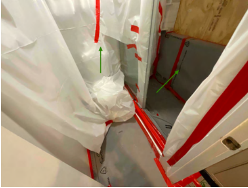
Photo 9 Unit No. 200 - View of protection installed at bathroom.
