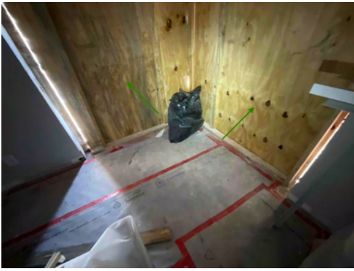
Photo 7 Unit No. 200 - View of corner window removed.
