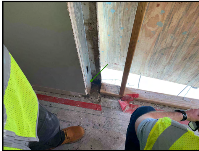
FIGURE 9 - Unit No. 200 - View of metal framing moved inwards for window installation.
