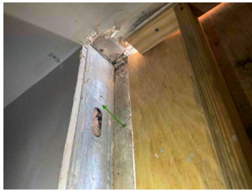
Photo 4 Unit No. 200 - View of metal framing moved inwards for window installation.
