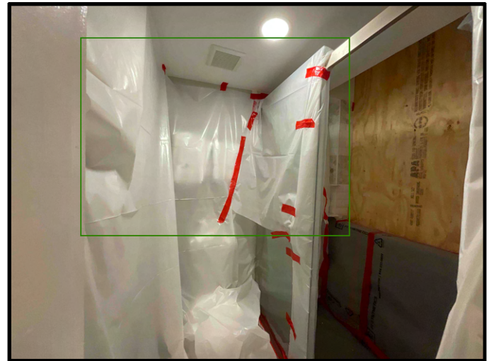
FIGURE 6 - Unit No. 200 - View of protection installed at bathroom.
