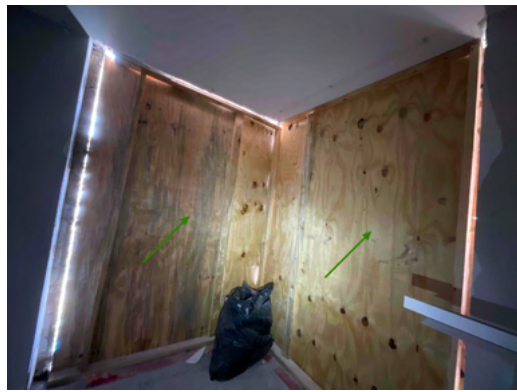
Photo 8 Unit No. 200 - View of corner window removed.
