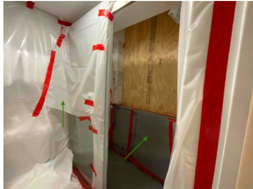
Photo 10 Unit No. 200 - View of protection installed at bathroom.
