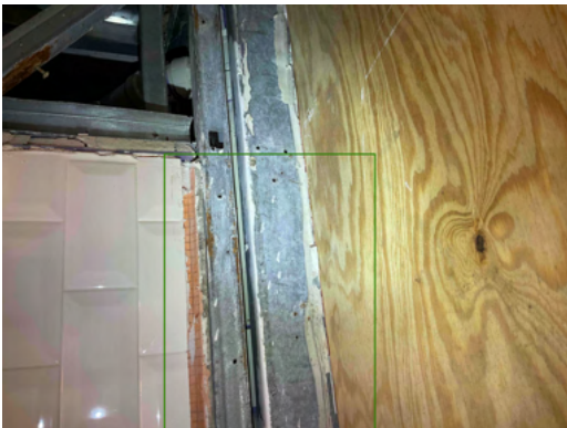
Photo 17 Unit No. 200 - View of existing tile removed from rough opening.
