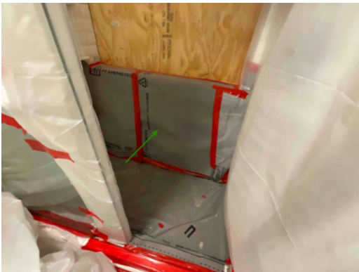
Photo 11 Unit No. 200 - View of protection installed at bathroom.
