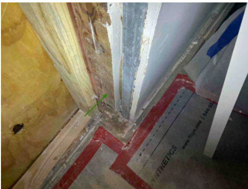
Photo 5 Unit No. 200 - View of wood bucking at West Jamb.
