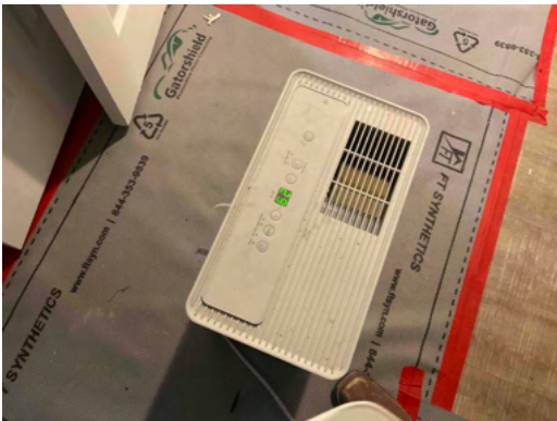
Photo 23 Unit No. 200 - View of dehumidifier running inside unit during window replacement.
