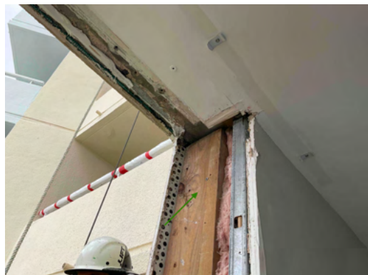
Photo 18 Unit No. 200 - View of wood bucking at West Jamb.
