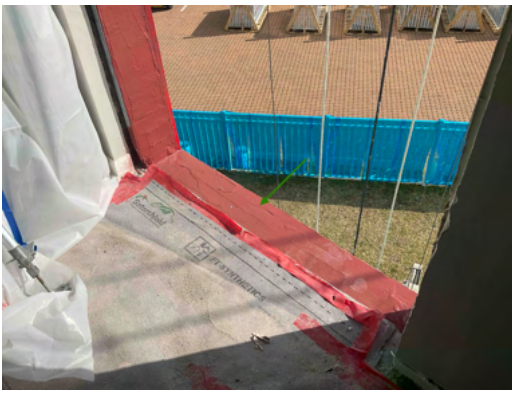
Photo 13 Unit No. 200 - View of new FastFlash waterproofing installed at rough opening.
