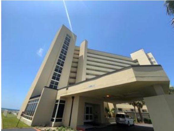
Photo 1 Perdido Sun – Overall view.
