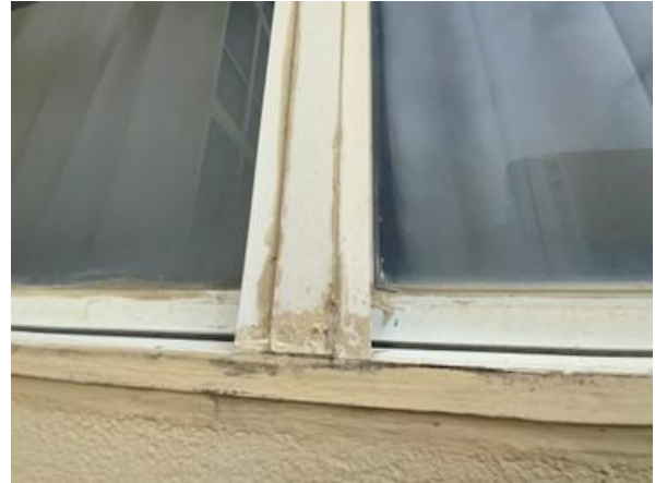
Photo 4 South Elevation – Overall view of windows – Typical.
